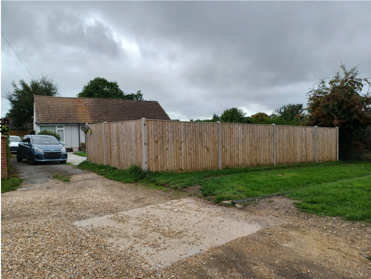
View of the site
